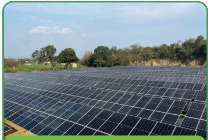
1.7 MW HPCL YEDIYUR CHAKENAHALLI, KARNATAKA
