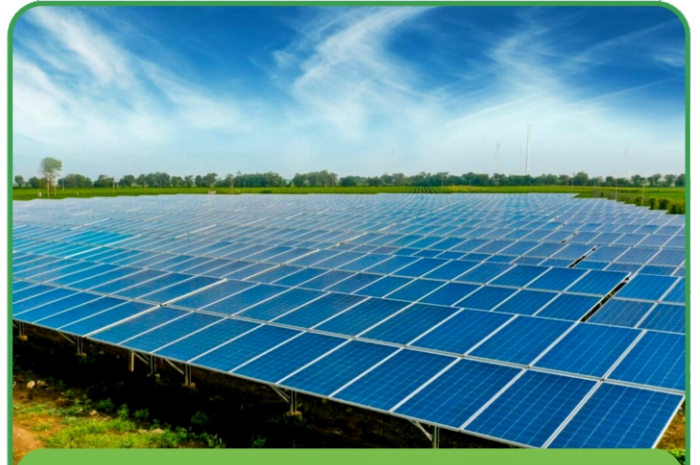
1.9 MW RAMPURA, GUJARA
